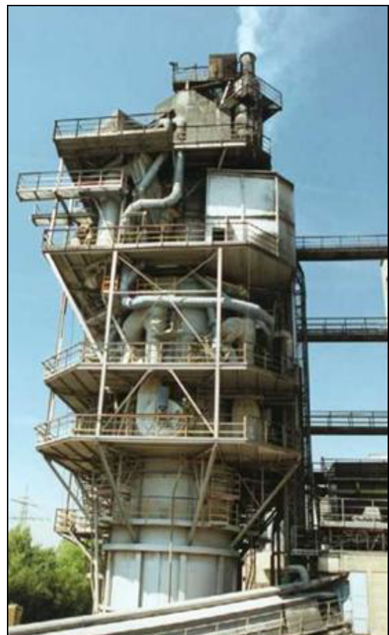
Figure 2.26: Example of an annular shaft kiln used in lime manufacture [44, EuLA, 2006]
