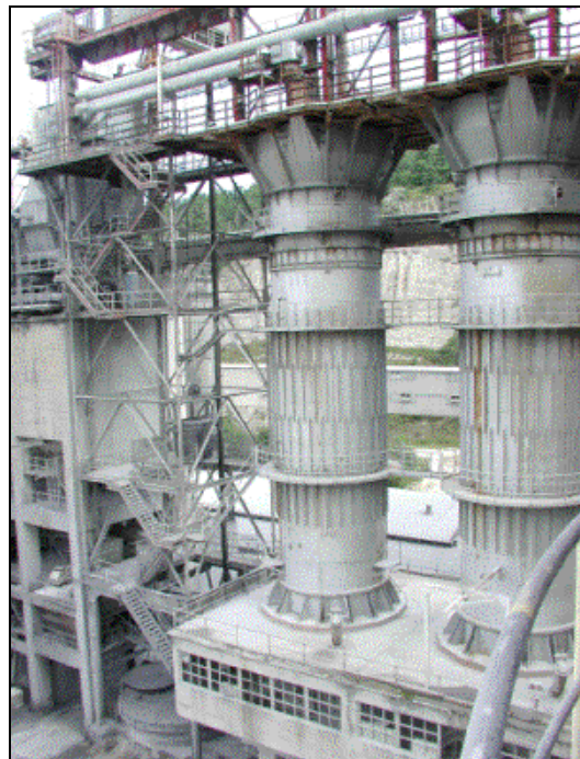
Figure 2.21: Mixed feed shaft kiln [44, EuLA, 2006]
